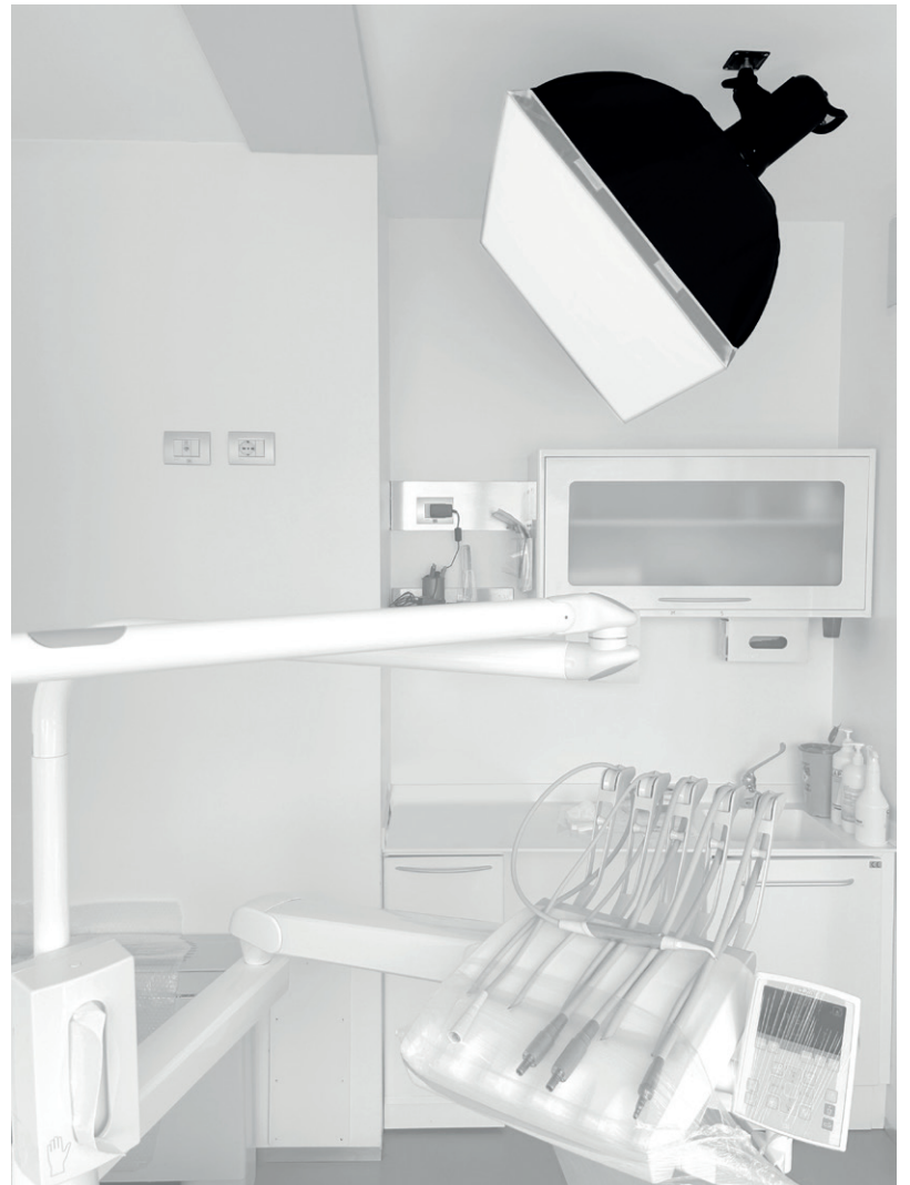
SOFT BOX ceiling installation
